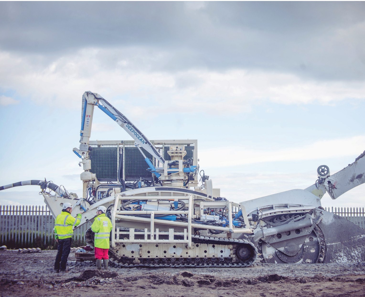
▲ Trenching vehicle trials, as part of a major upgrade project
